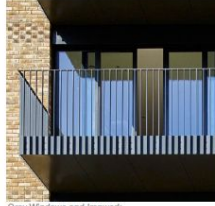
Grey Windows and Ironwork
